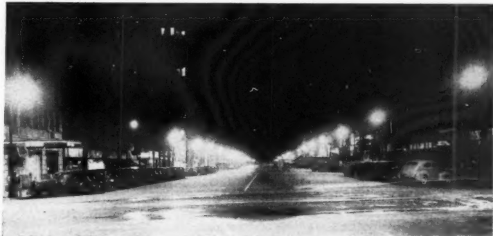
The outstanding feature of Chattanooga's new street lighting system is the use of 80 pendant mercury-incandescent luminaires in the downtown area. Developed by General Electric engineers, each luminaire operates two 300-watt incandescent lamps and one 400-watt mercury lamp. The luminaires are spaced 100 feet apart and opposite one another on both sides of the street. This night picture was taken along Broad Street.
